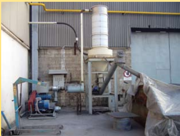
Central vacuum system for calamine in electrorodes manufacturer
