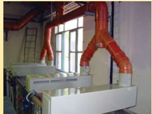
Special plastic suction hoods and ducts
