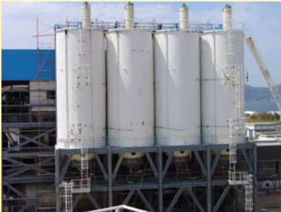
Silo equipment for dried sludge silos at Athens municipality
