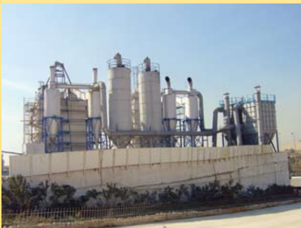
De-dusting of 3 lime stone furnaces 120 tn/h each
